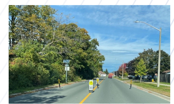
Vertical Centreline Treatment
