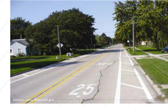
Pavement Marking Signs
